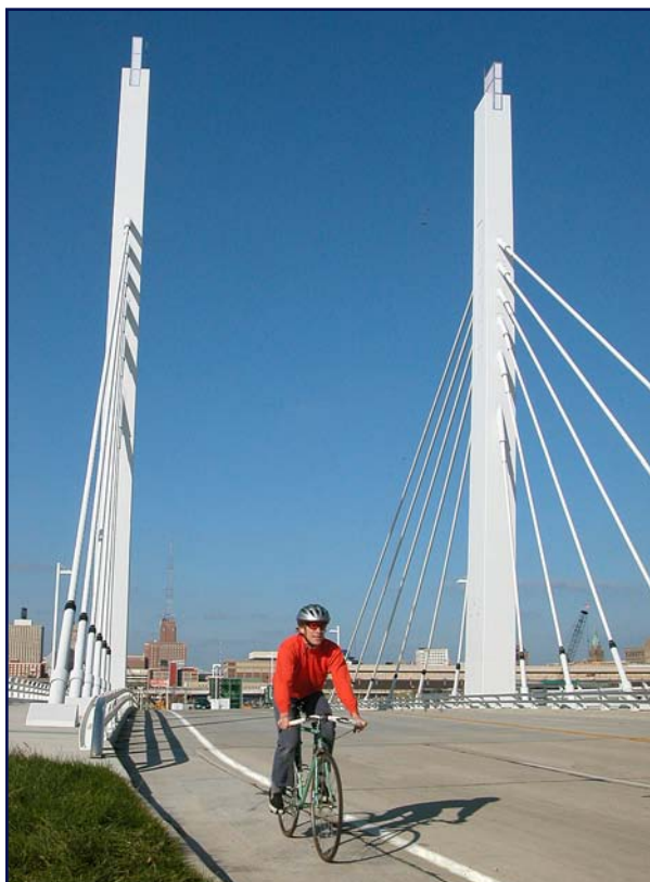
6th Street Bridge
