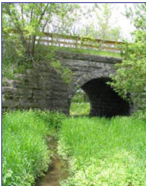
Bridge on the Eisenbahn Bike Trail near West Bend
