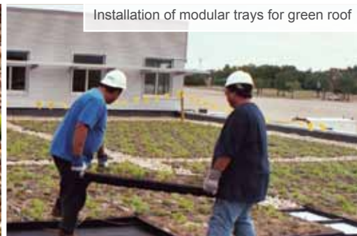
Installation of modular trays for green roof
