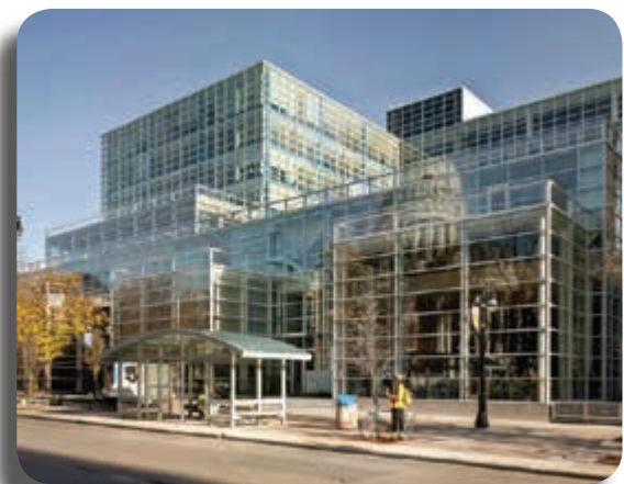
Madison’s US Bank Plaza recently received LEED Gold certification. Home to Graze and L’Etoile, two of Madison’s sustainable food restaurant pioneers. Image courtesy of Urban Land Interests.
