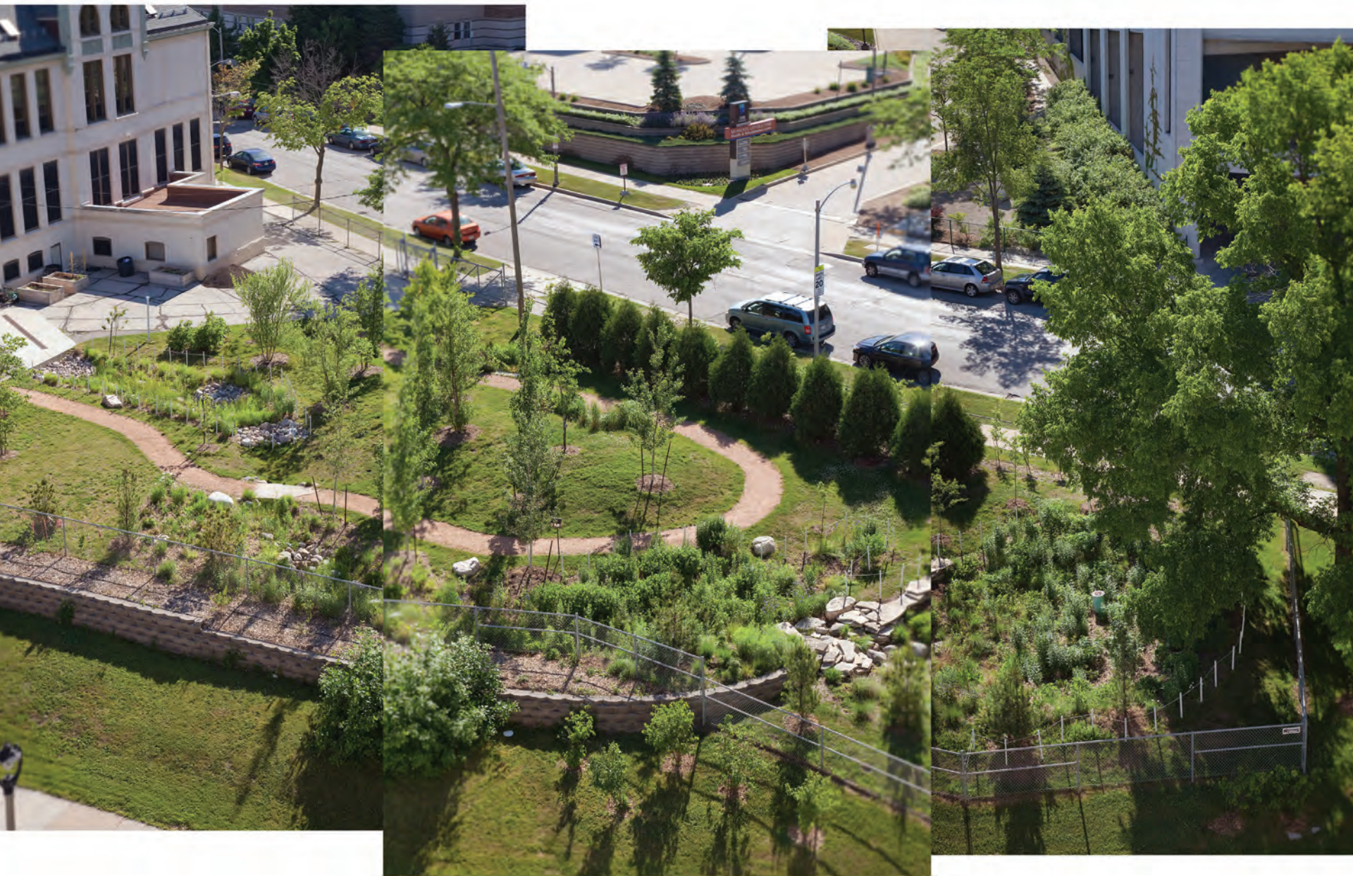
Maryland Avenue Montessori School rain garden, Milwaukee
