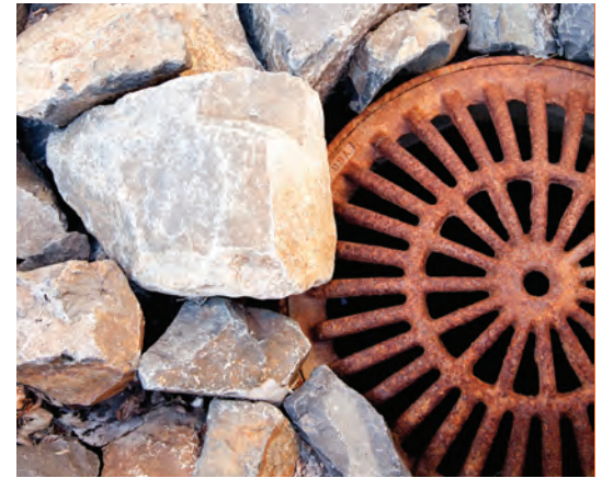
The Brewery, infiltration trench, Milwaukee
